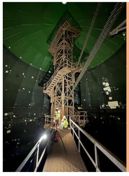
Structural assessments are ongoing for a spiral staircase that is unique to Tank 6. Its removal is required for safe tank cleaning.
