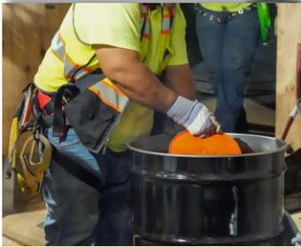
Sludge is placed into 55-gallon drums that are then sealed.
