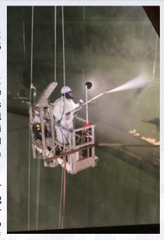
the discharged wash water from the tank show it consists of approximately 1% residual fuel and 99% wash water, which includes the cleaning agent.
