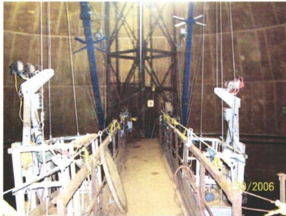
VIEW FROM MANWAY INTO TANK AFTER CLEANING COMPLETED SUSPENDED SCAFFOLDING SYSTEM STILL IN PLACE
